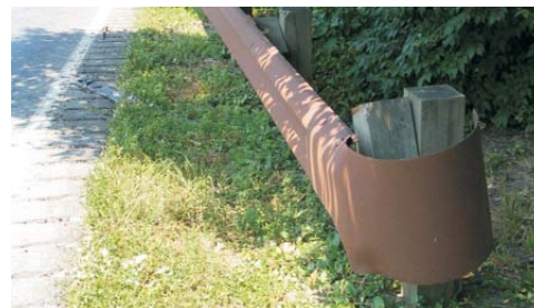
Cor-Ten Guard Rail with Wood Post River Road
